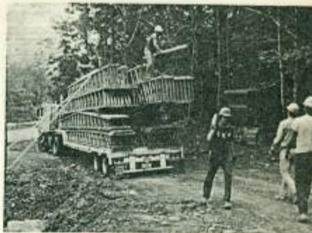
Unloading trusses for the new house.
